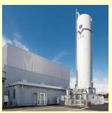
By integrating storage tanks, vaporizers and other equipment, the space necessary is significantly reduced and maintenance is simplified. By converting fuels from petroleum and coal to LNG, CO<sub>2</sub> emissions are reduced.
