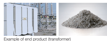
Example of end product (transformer)
