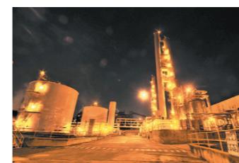
On-site gas supply for steelmakers (India)
