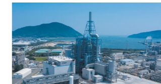
Woody biomass and coal co-fired power generation Generation capacity: approx. 112,000 kW (Began operations in July 2019)
