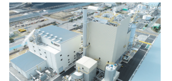
Woody biomass mono-fired power generation Generation capacity: approx. 75,000 kW (Began operations in April 2021)
