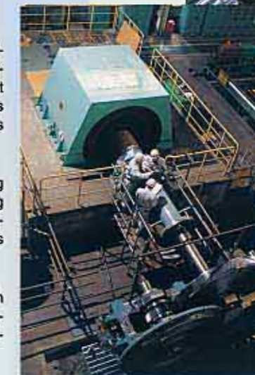
Compressor disassembly and maintenance
