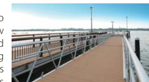
Example of ECOROCA® construction at Koshigaya Lake-Town
