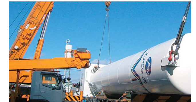
V1 facility construction
