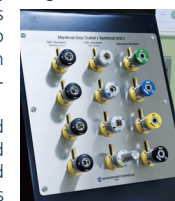
Medical gas piping outlet
