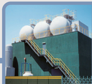
The No. 1 oxygen PSA installation geared towards electric furnace manufacturers. A forerunner of Air Water's "total gas solutions" system.
