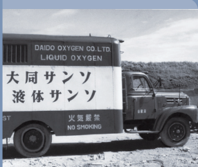
Daido Sanso's oldest liquid oxygen tank truck. Liquid oxygen was sold directly from a two-ton tank.
