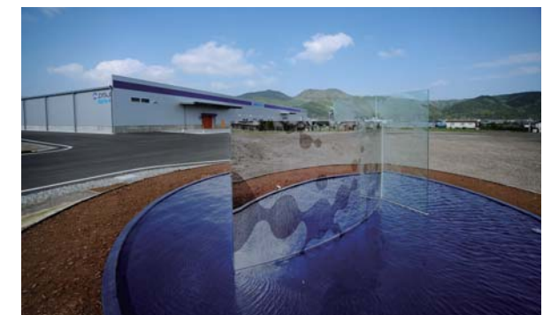
AW-Water Shinano-omachi Plant and "Air & Water Circulation" monument
