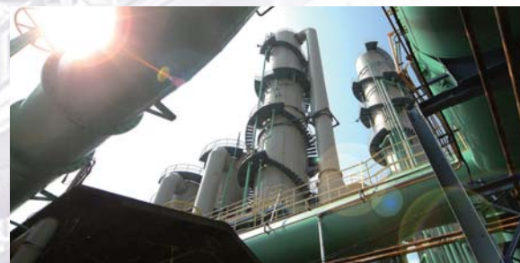
Gas purification plant in Wakayama Plant
