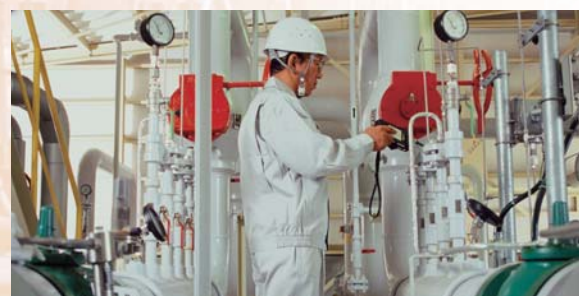
Chitose Pipeline Distribution Center
