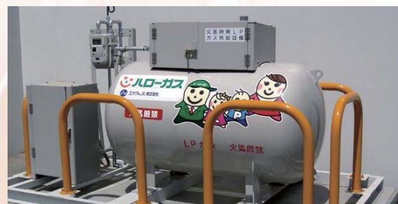
LP gas supply equipment for use in disasters
