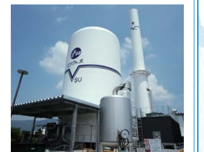
VSU in Hofu Plant
