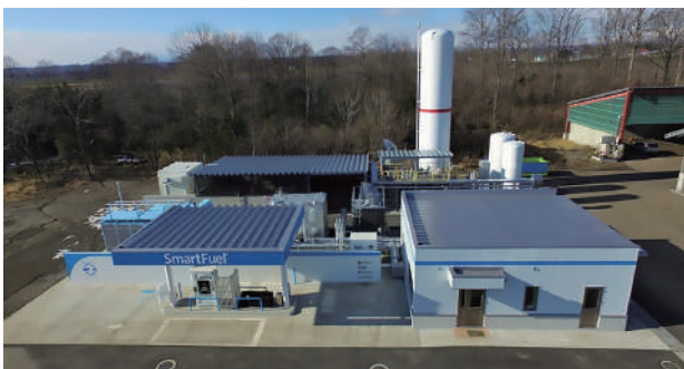
A hydrogen farm in Shikaoi, Hokkaido
