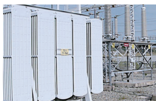
Example of end product (transformer)
