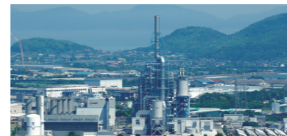
Woody biomass and coal co-fired power generation Generation capacity: approx. 112,000 kW (Began operations in July 2019)
