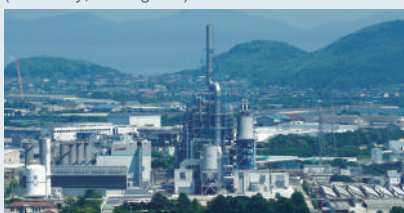
Woody biomass and coal co-fired power generation Generation capacity: approx. 112,000 kW (Began operations in July 2019)
