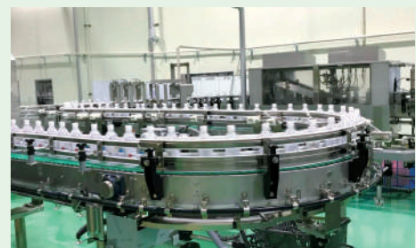
New plastic bottle-filling line at the Hokkaido Eniwa Plant
