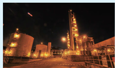
The industrial gas business in India we acquired in July 2019 (on-site supply for the Jamshedpur steelmaking plant)
