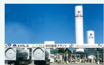
Liquefied biomethane production plant
