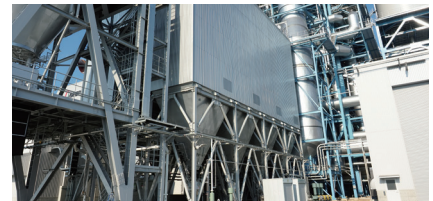
Bag filters remove hazardous substances from the boiler's combustion gases
