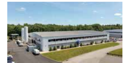
American Gas Products plant
