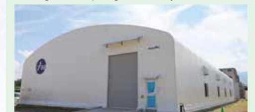
Onshore aquaculture plant
