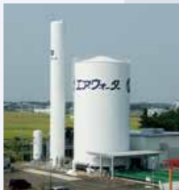
The first VSU, Niigata Ekisan
