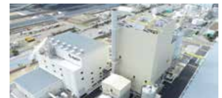
Wood biomass power generation
