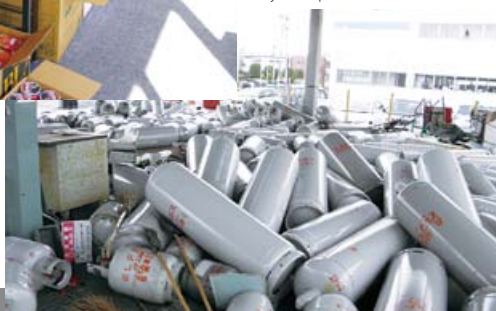
A scene at the Sendai Office's LP gas filling site immediately following the earthquake. All the site's gas cylinders were toppled by the quake.
