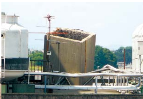
A collapsed chimney at a hospital in Sukagawa City, Fukushima
