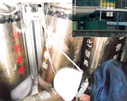
Work being carried out to secure gas cylinders knocked over by the earthquake
