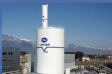
High-efficiency compact liquid nitrogen/oxygen co-production plant (VSU)
