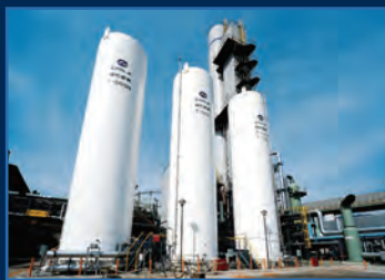
Large-scale cryogenic air separation system
