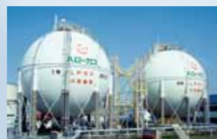
Hello Gas spherical tanks (secondary station)
