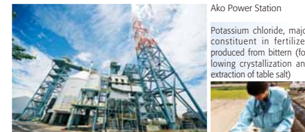
Ako Power Station
