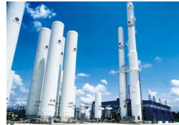
System for stable oxygen supply to meet demand fluctuation (at Air Water Vietnam)
