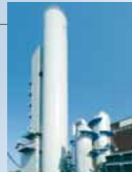
Large scale on-site plant
