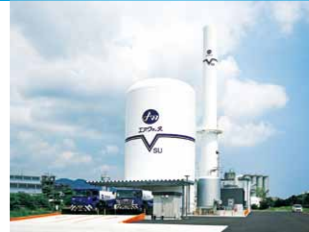
Air Water's 11th VSU facility, in Hofu. Enabling locally-sourced industrial gas distribution systems.
