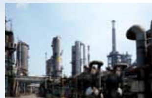
Gas purification plant
