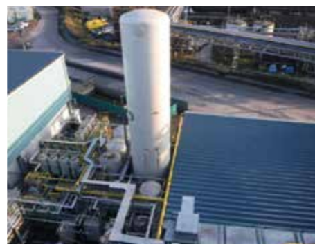
COURSE50 Blast furnace gas purification facility
