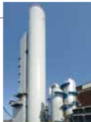
Large scale on-site plant
