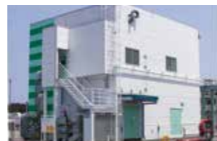
GMP plant for high-active chemicals
