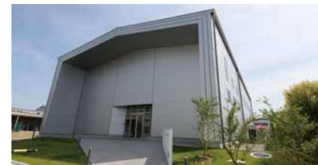
Vibration Test Center newly established on the premises of the factory of Air Water Safety Service head office
