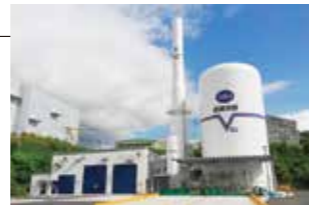
Compact, high-efficiency liquid nitrogen/oxygen co-production plant "VSU"
