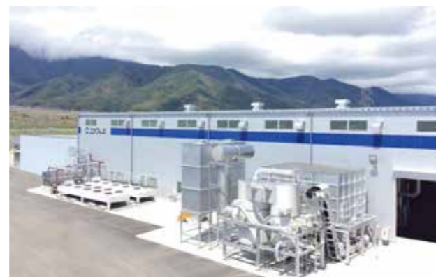
An external view of the Azumino Biomass Energy Center
