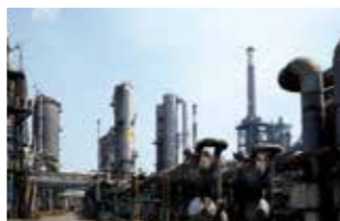
Gas purification plant
