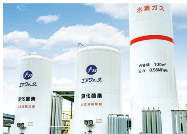
Manufactured hydrogen storage tank (right) and tanks of liquefied nitrogen and liquefied oxygen used in manufacturing (left and center)
