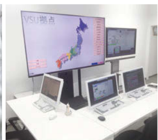
Remote Monitoring & Support Center
