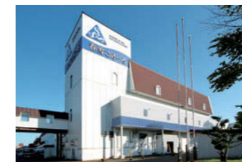
Saveur SS Hayakita Plant
