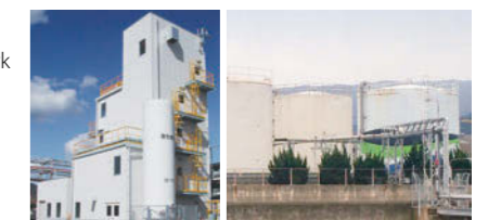
Hydrogen selenide manufacturing equipment Imari Logistics Base
