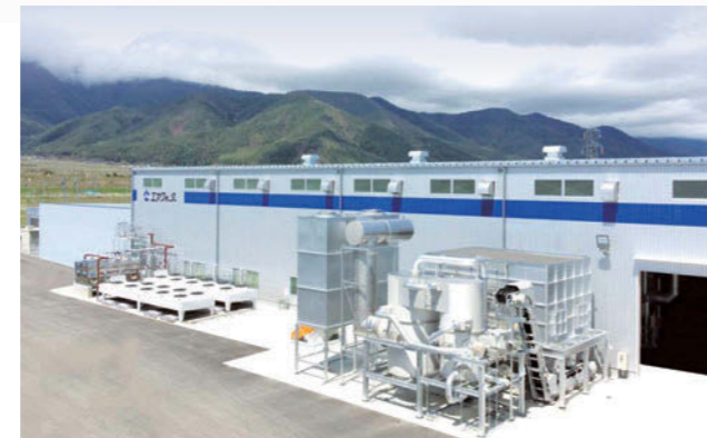
Biomass Energy Center
