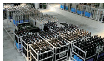
High-pressure gas filling station
