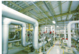
Supplying natural gas via pipeline
