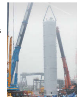
Construction of Air Water Carbonic Inc. Kawasaki Plant
