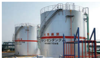
Crude benzene tank
