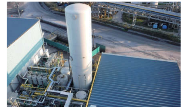
COURSE50 blast furnace gas purifying facility
