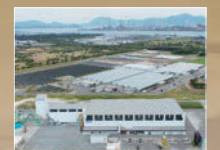
Tateho Chemical Industries' Hibikinada plant
