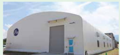
Onshore aquaculture plant
