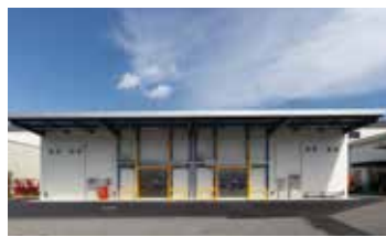
Hazardous material storage
