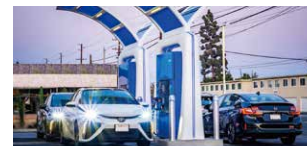
FEF's hydrogen station
