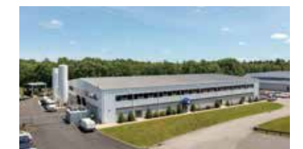
American Gas Products plant
