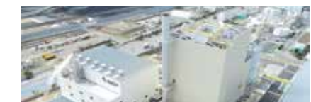
Wood biomass power generation
