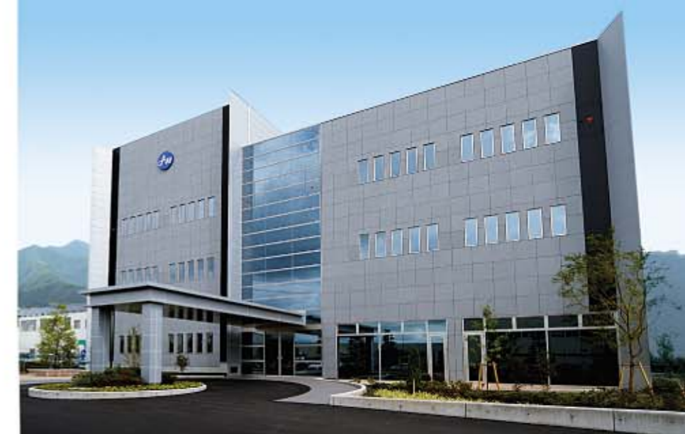
New Research & Development Institute (on the banks of the Azusa River in Matsumoto City, Nagano Prefecture)
